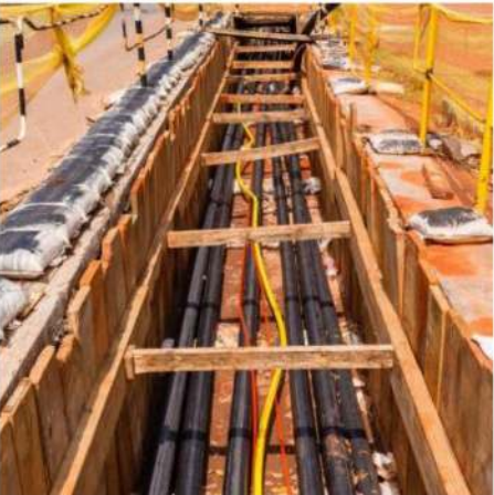
Both of the images above show how various utility lines can be safely co-located underground along thoroughfare rights of way.
