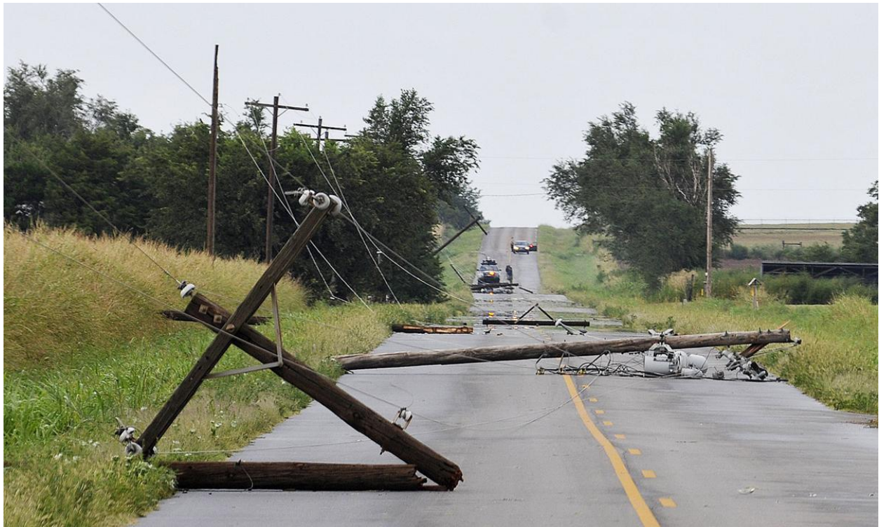
Figure 2 - Downed utility poles obstruct Oakwood Road following a thunderstorm.
