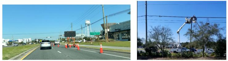
Construction crews have installed signage (above), removed street lights (right), and have begun clearing areas for pipe installation. Below is a rendering of an underpass entry.
