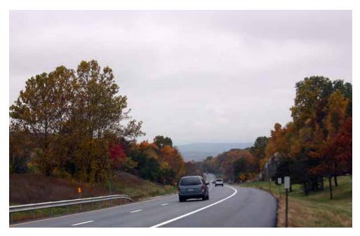
Interstate 84 running east-west just above New York City is a heavily traveled route used by trucks and autos, and it is fairly typical of all of New York's interstates and freeways. Completely, or relatively free of billboards, screened from adjacent commercial uses, and sensitively integrated into the topography with long, sweeping curves and variable medians, these highways are *Integrated Freeways* built to interstate standards.
