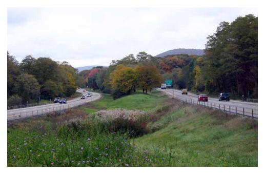
Sensitive design of highways is a complex and demanding discipline. The objective is a continuous physical and visual flow of the alignment, integrated with the topography and landscape. That usually means a high ratio of curves to tangents, careful merging of horizontal and vertical curves including spiral transitions, and variable medians that acknowledge and celebrate topographic changes, vegetation, water features, and geological formations.
