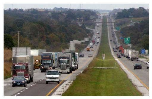
A section of I-70 typical in two ways – a rigid straight line alignment (this section running just south of Booneville stretches 21 miles without a curve!) and an over-abundance of trucks. On the other hand, this photo is a very rare short stretch that is relatively free of billboards.
