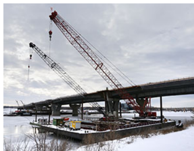
Scenic America, a group that opposes digital highway billboards, says it cost the state $4.3 million to remove a digital billboard as part of the Lafayette Bridge project over the Mississippi River in St. Paul. (File photo: Bill Klotz)
